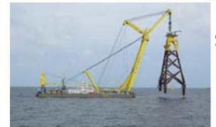
Jacket installation using a floating vessel
