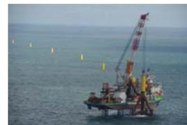
Tripod installation using a jack-up vessel
