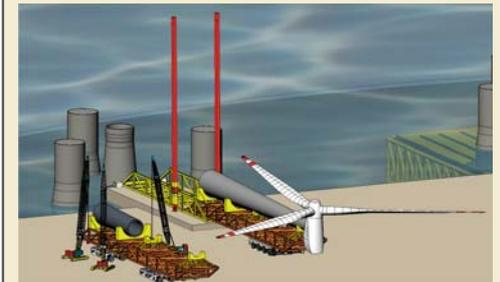
The substructure is towed into position, and grounded (by ballasting) onto supports to eliminate the typical challenge of relative motion between substructure and lifting arrangement.
