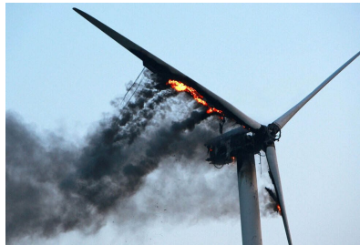
Figure: Wind Turbine on fire. 1
