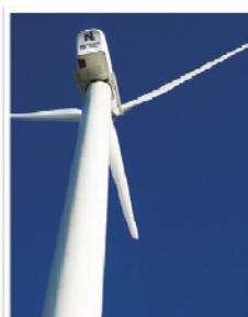
Example 100 kW turbine for 1/3 scale testing at UMaine Test Site deployment
