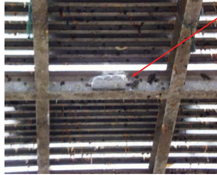
For corrosion protection, galvanic anodes are used. The need for galvanic anodes is ~10% of what is needed for steel structures.
