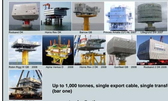
**Up to 1,000 tonnes, single export cable, single transformer (bar one)**
