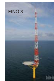
Measurements up to 100 m Shallow waters (~ 20 m)
