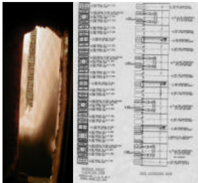
Figure 2: Burner assembly at the corner of a tangentially-fired boiler.
