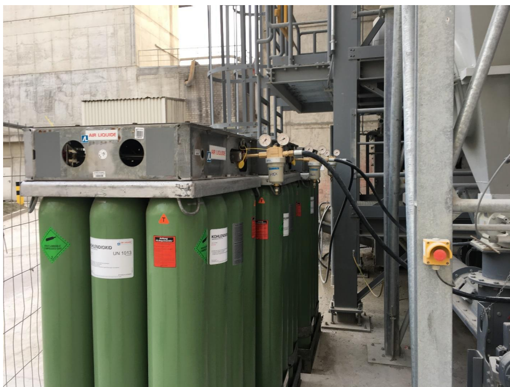
Figure 3.19: CO 2 gas filling station with 3 bundles, 12 bottles each
