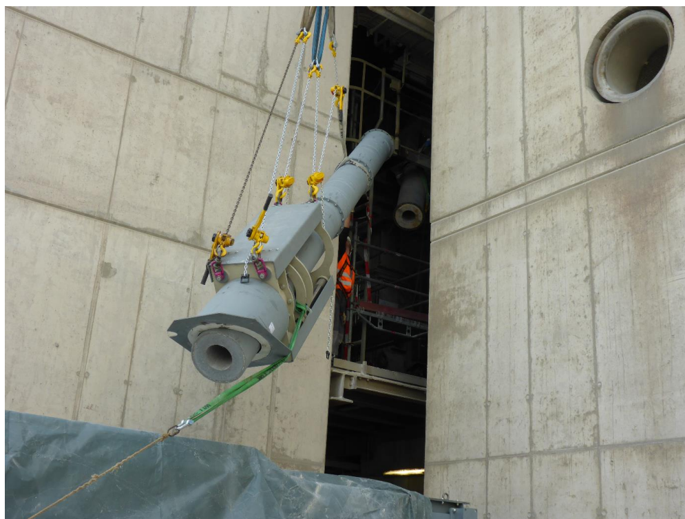
Figure 3.9: Installation of the hot clinker extraction device.
