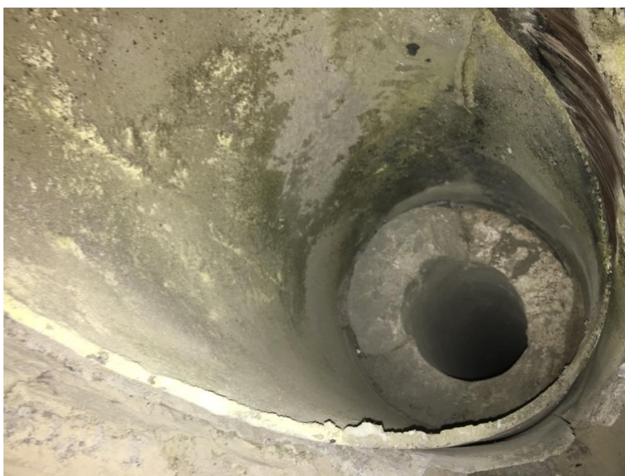
Figure 7.1: Hot clinker extraction tube during repair works after 2 nd damage
