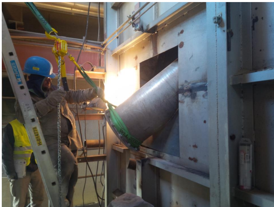
Figure 3.7: Installation of the adaption piece into the existing cooler front wall
