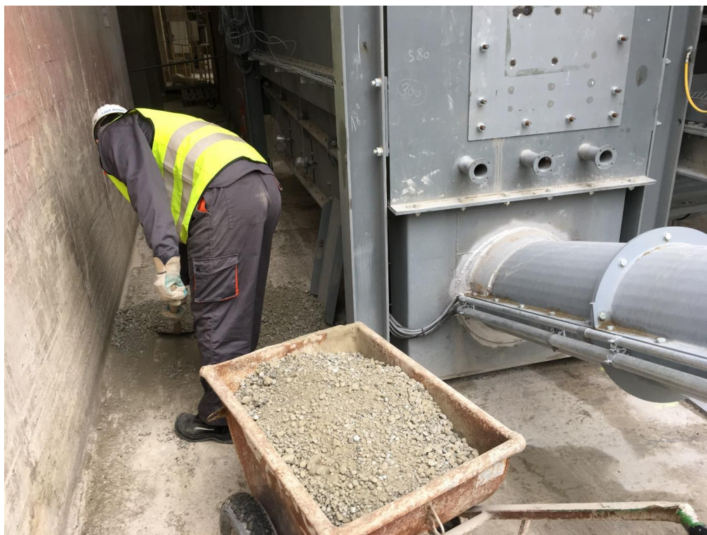
Figure 3.13: Functional test and cold commissioning of the cold clinker discharge screw conveyors
