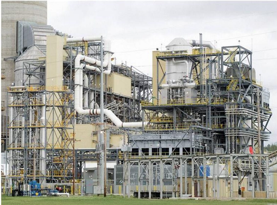
Figure 3: Mountaineer Product Validation Facility plant.
