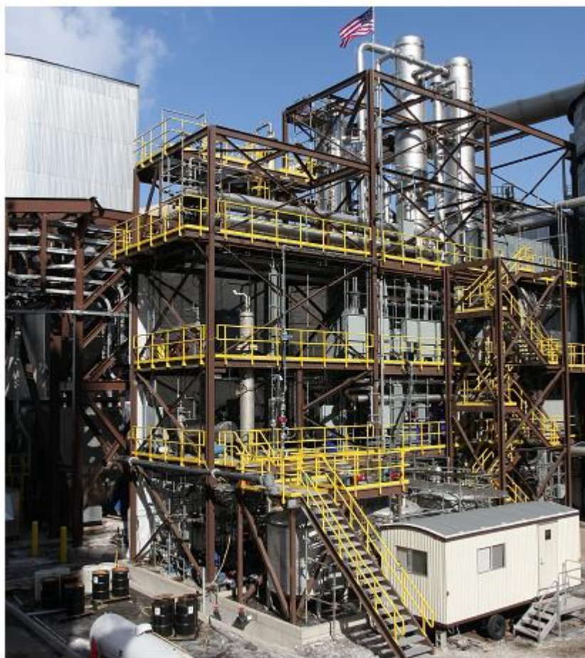
Figure 2: WE Energy pilot plant.
