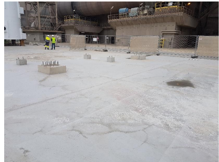
Slab completed (26 June 2018)
