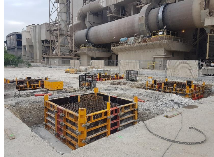
Piles ready for pouring (16 May 2018)
