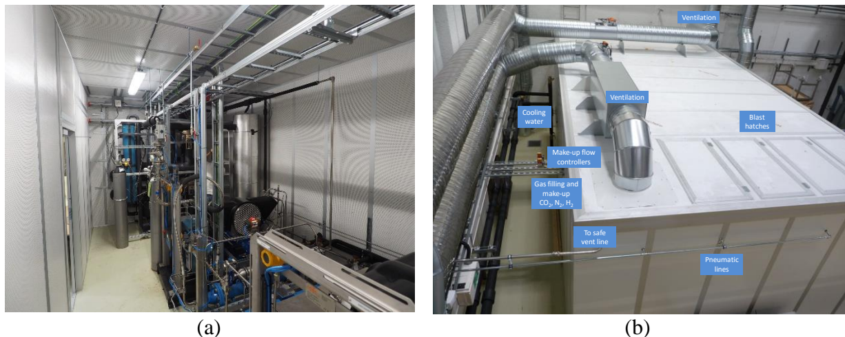
Figure 16. Interior (a) and exterior (b) of the low-temperature CO 2 liquefaction unit.
