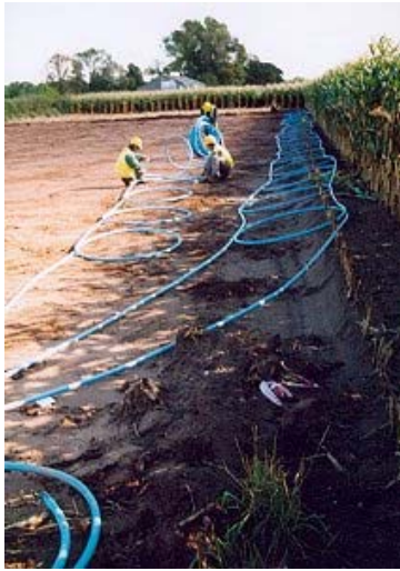
Figure 10.1: Slinky coils prior to installation
