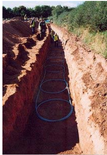
Figure 10.2: Slinky coils laid horizontally in trench
