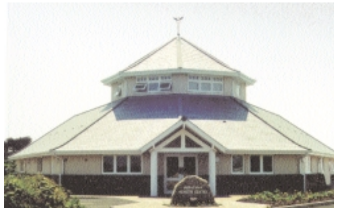
ABOVE The UK's first non-domestic GSHP installation is sited here, at a health centre on the Isles of Scilly GEOSCIENCE. TOP RIGHT Work on heat pump installation at a new IKEA distribution centre, Peterborough, UK. GEOSCIENCE FAR RIGHT End of double U-tube BHE GEOWATT
