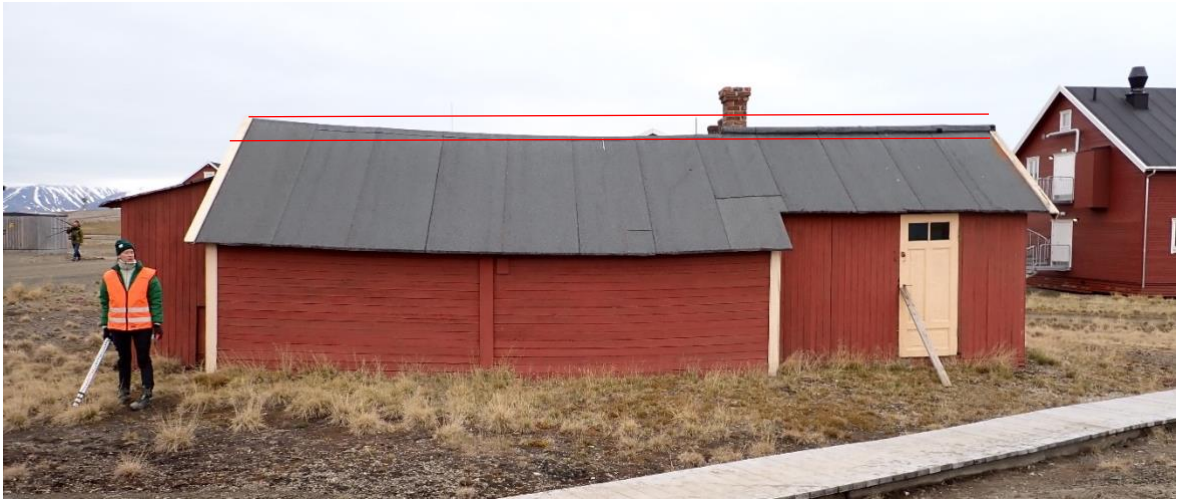
Figure 10. Differential settlements of Green Harbour House in Ny-Ålesund, June 23, 2023. Photo by Anatoly Sinitsyn/SINTEF.
