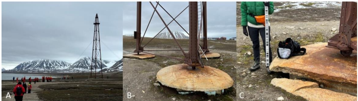
Figure 11. Terrain settlements at Luftskipsmasta, June 26, 2023. Photo by Anatoly Sinitsyn/SINTEF.
