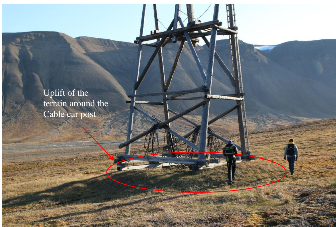
Figure 23. Post Nr. 6 at the Cable car line 5. This post is resting on a small bump/hill that is probably created as a result of frost heave, which is stimulated by absence of snow in winter, September 3, 2021. Photo by Anatoly Sinitsyn/SINTEF.
