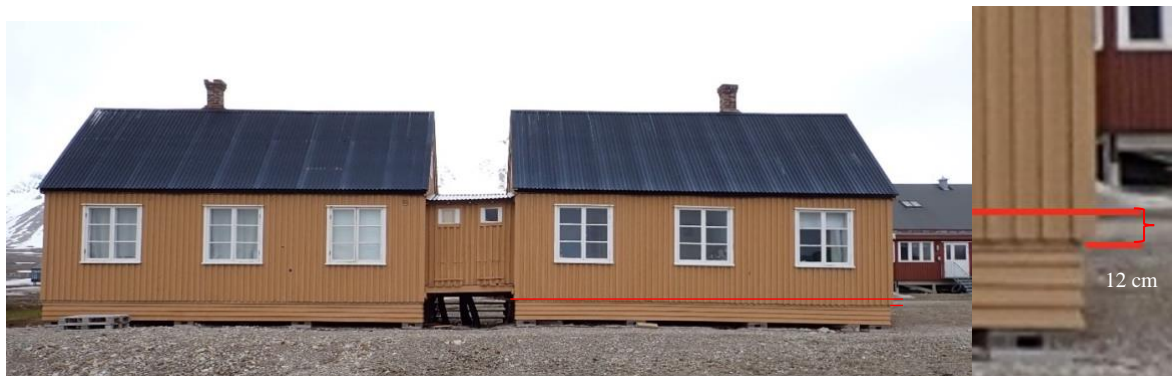
Figure 9. Settlement at London houses in Ny-Ålesund. Photo by Anatoly Sinitsyn/SINTEF.
