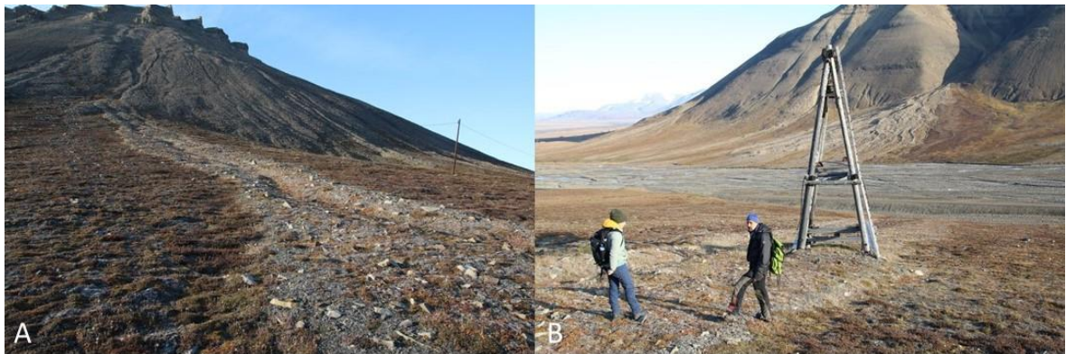
Figure 12. Post nr. 9 at the Cable car line 5 that has survived a debris flow, September 3, 2021. Photos by Anatoly Sinitsyn/SINTEF.
