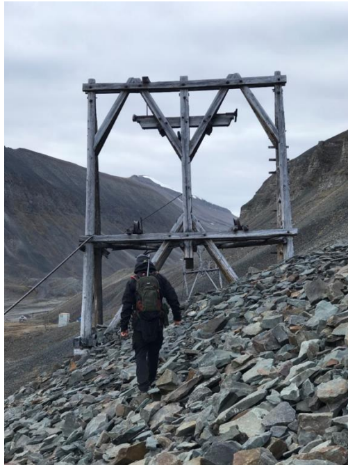
Figure 21. Accumulation of rock debris at cableway trestle Nr. 5, Line 1b as an indicator of previous snow avalanche activity in the area. Despite impacts from snow avalanches and structural damages (one broken foundation) Cableway trestle Nr. 5 is still standing.
