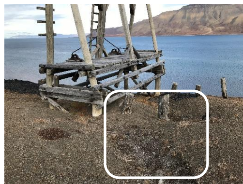
Figure 37. Cableway post Nr. 15 on the Line 3, seasonal creek running under the structure (close look-up). White rectangle depicts the creek.
