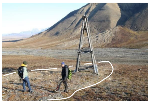
Figure 20. Remains of old debris flow at cableway trestle Nr. 9, Line 5. White line presents outline of debris flow.
