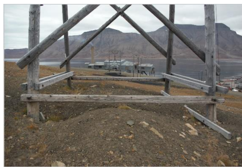
Figure 24. Ground depressions under cableway trestle Nr. 23 on the Line 1b (2021). This trestle was restored in 2007. Picture: © Snaprud Christensen, C.
