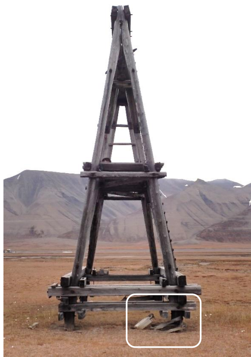
Figure 3. Broken cross-bracing element at cableway trestle Nr. 36 at the Line 6 (general view).
