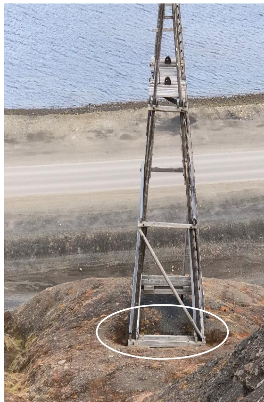
Figure 15. Cableway Nr. 18, Line 3 – terrain settlements under and around the structure. White line outlines settled area.
