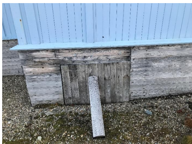
Figure 89. Opening is the "skirt" of Telegrafan, Ny-Ålesund. Such opening should be kept open during winter and closed during summer.
