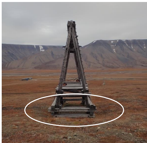
Figure 14. Settlement of terrain due to permafrost degradation and large uniform settlement of Cableway post Nr. 21 at the Line 6 into the permafrost. White line outlines settled area.
