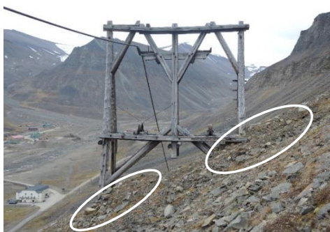
Figure 45. Accumulation of rock debris at cableway trestle 10, Line 1b. Accumulated material around the structure is marked with ovals.
