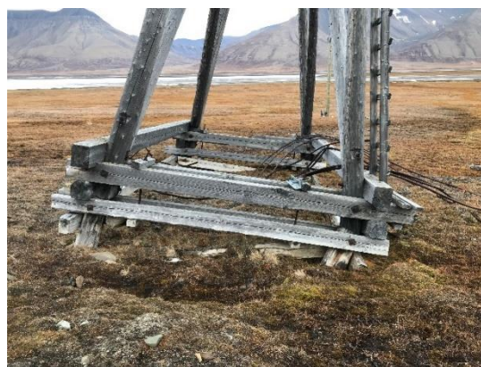
Figure 13. Cableway post nr. 41 at the Line 5-6 – large vertical settlements and uneven tilt (close look-up).
