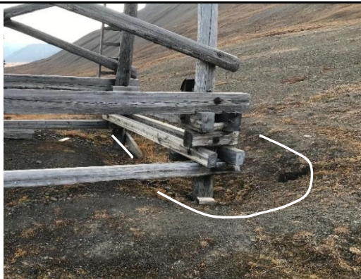
Figure 27. Depressions around vertical foundation elements at cableway trestle Nr. 19 at the Line 5-6.
