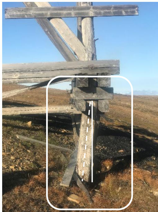
Figure 2. Cableway post Nr. 15 on the Line 5-6, tilt of foundations due to solifluction (close look-up).
