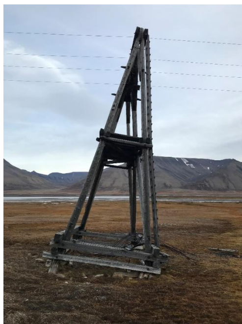
Figure 12. Cableway post nr. 41 at the Line 5-6 – large vertical settlements and tilt due to degradation of permafrost (general view).
