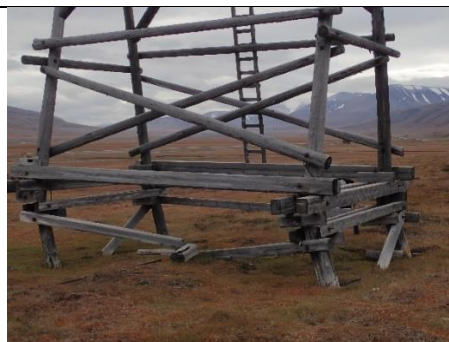
Figure 44. Heavy tilt of vertical foundation elements of the cableway trestle Nr. 17 at the Line 6. Tilt of foundation elements occurs due to action of solifluction.
