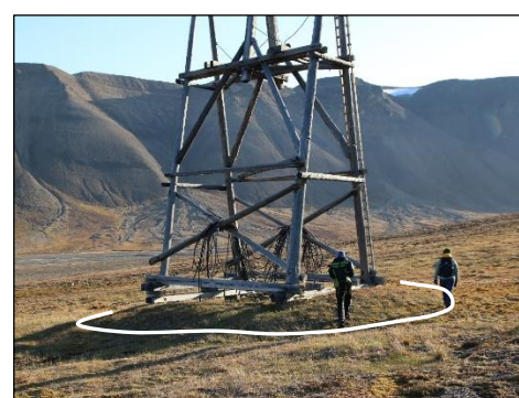
Figure 39. Cableway trestle Nr. 16, Line 5: ground is elevated in relation to surrounding tundra. White line presents outline of the elevated terrain.
