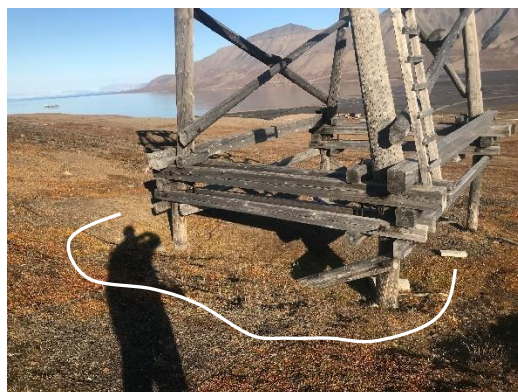
Figure 28. Depressions around vertical foundation elements at cableway trestle Nr. 20 at the Line 5-6.
