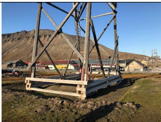
Figure 25. Ununiform ground settlements below recently restored cableway trestle Nr. 6 at the Line 5-6. One shall acknowledge that some uneven terrain below the object is due to the excavation activities.
