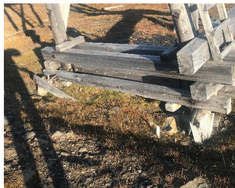
Figure 11. Tilt of the Cableway post nr. 16 on the Line 5-6 due to rapture of foundation element (close look-up).
