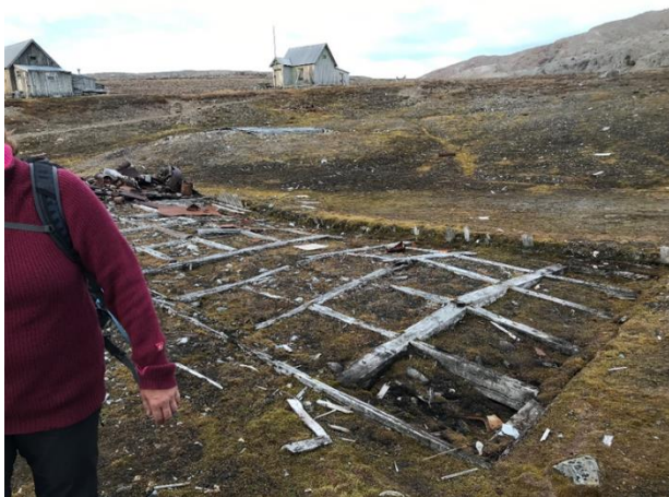
Figure 67. Foundation remains in Ny-London (2021), similar foundation type is believed to be used at Green Harbour House.
