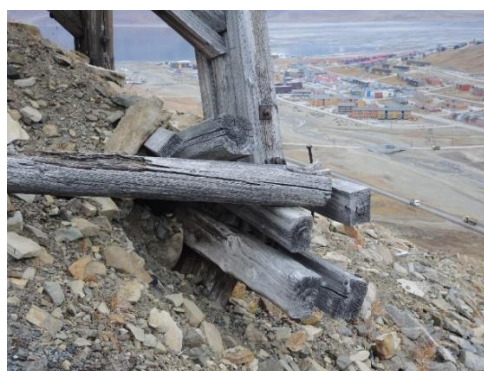
Figure 46. Close-up at accumulated material at cableway trestle Nr. 10, Line 1b.
