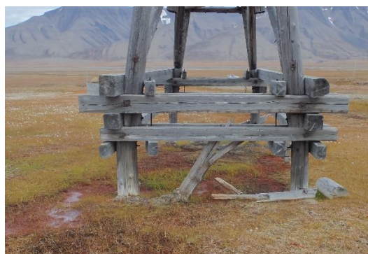
Figure 4. Rupture of cross-bracing element at cableway trestle Nr. 25, Line 6.
