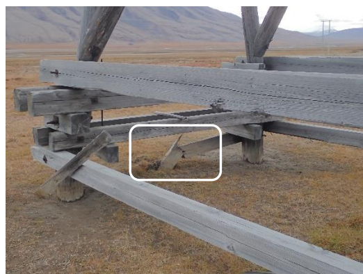
Figure 5. Broken cross-bracing element at cableway trestle Nr. 36 at the Line 6 (close look-up).
