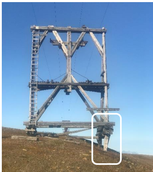
Figure 1. Cableway post Nr. 15 on the Line 5-6, tilt of foundations due to solifluction (general view from the front).
