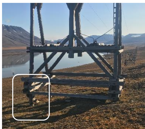
Figure 8. Cableway post nr 22 on the Line 5-6, rupture of foundation element above the ground, presumably due to rot (general view from the front).
