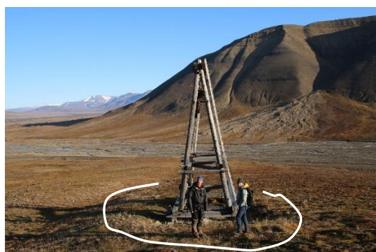
Figure 38. Cableway trestle Nr. 10, Line 5: ground under the structure is elevated in relation to surrounding tundra, while the structure seems to be settled into the terrain. White line presents outline of the elevated terrain.
