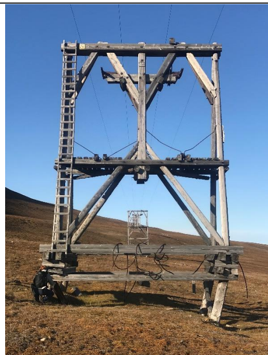
Figure 50. Effects of solifluction on foundation of cableway trestle Nr. 26 at the Line 5-6: heavily tilted foundations.
