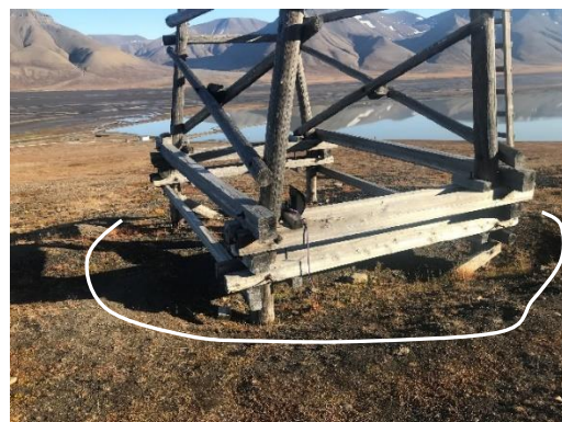
Figure 34. "Slide-like" settlements of the ground around structures on sloping terrain – Cableway post Nr. 19, Line 5-6 (close look-up). White line depicts "scar" of the "slide".
