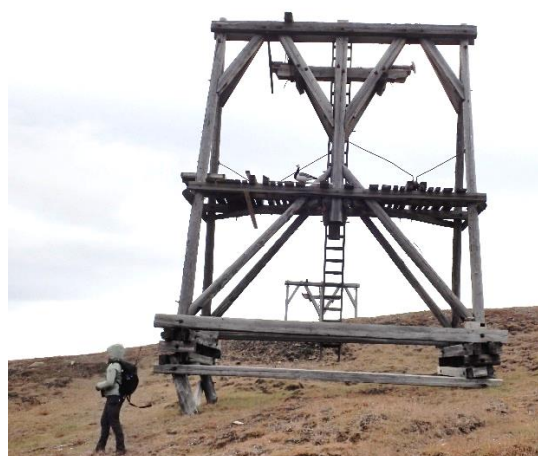
Figure 7. Heavy tilt of two foundations of the cableway post Nr.22 on the Line 5-6.
