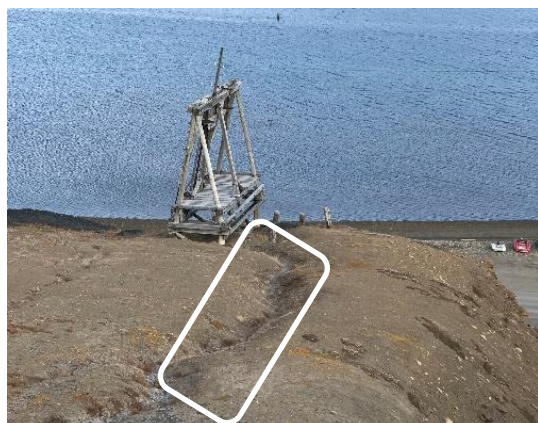
Figure 36. Cableway post Nr. 15 on the Line 3, seasonal creek running under the structure. Creek may cause both, surface erosion under the structure and increased degradation of permafrost. White rectangle depicts the creek.
