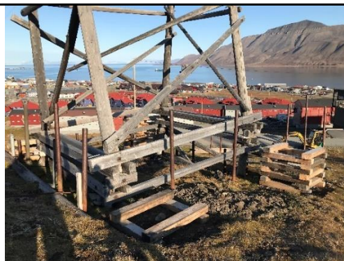
Figure 42. Cableway trestle Nr. 8 at the Line 5-6. This structure was affected by solifluction, and an attempt to stop this process was undertaken some years, see rusty metal poles.
