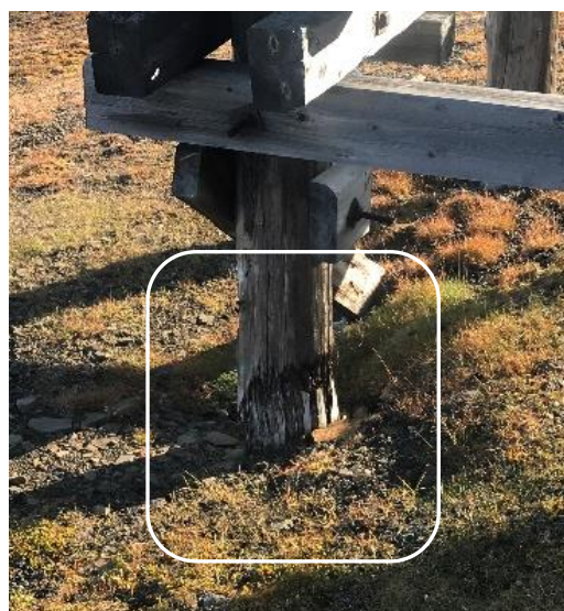
Figure 9. Cableway post nr 22 on the Line 5-6, rupture of foundation element above the ground, presumably due to rot (close lookup).
