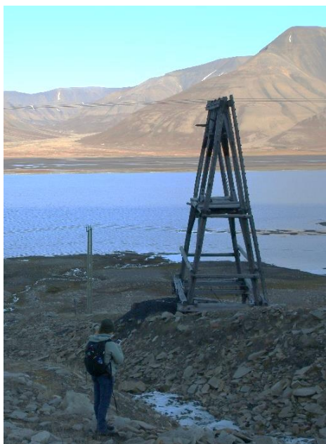
Figure 51. Development of a ravine next to cableway trestle Nr. 36, Line 5-6. This development of ravine may lead to local slide of the slope supporting the trestle and subsequent collapse of it.
