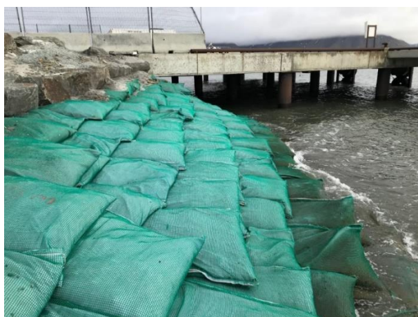
Figure 92. Example of revetment form geotextile bags (Svea, Svalbard).
