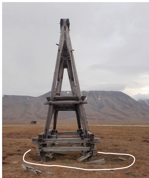
Figure 17. Cableway trestle Nr. 9, Line 6: massive terrain settlements under and around the structure and rupture of cross-bracing element. White line outlines settled area.
