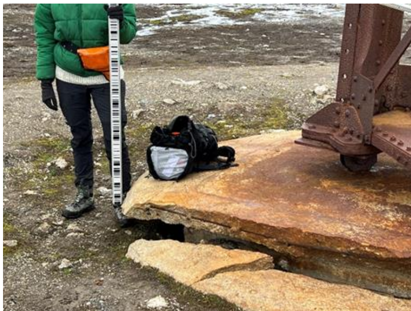
Figure 79. Terrain settlements (about 30-40 cm) around Luftskipsmasta (picture: 2022).
