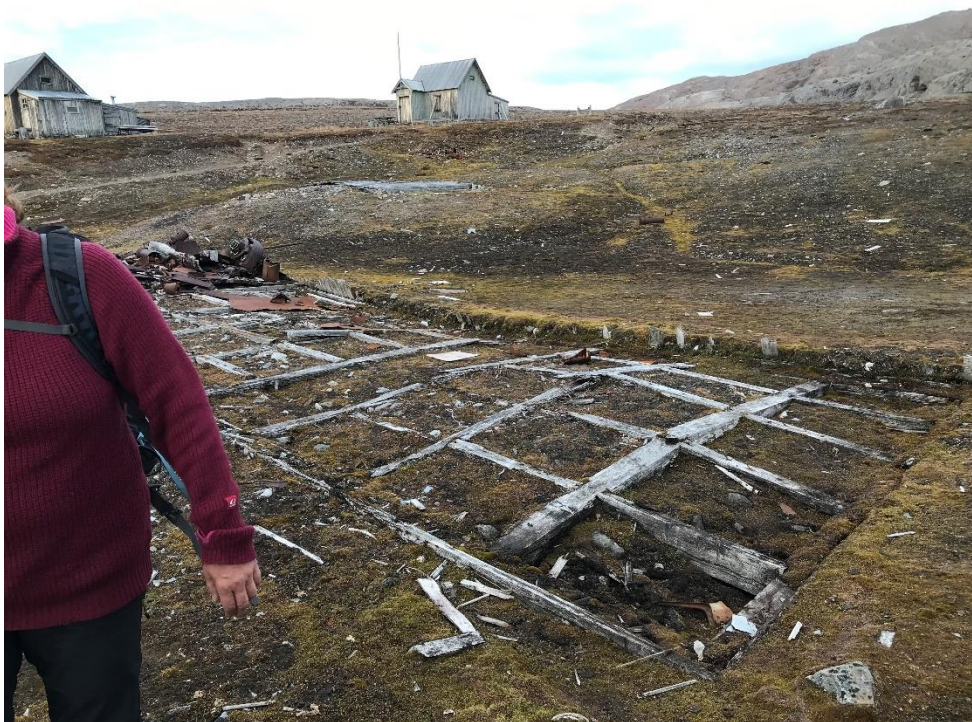
Figure 13: Foundation remains in Ny-London (2021), similar foundation type is believed to be used at Green Harbour House. Picture: © Anatoly Sinitsyn/SINTEF AS.
