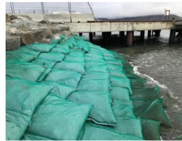
Figure 1. Example of revetment form geotextile bags (Svea, Svalbard).
