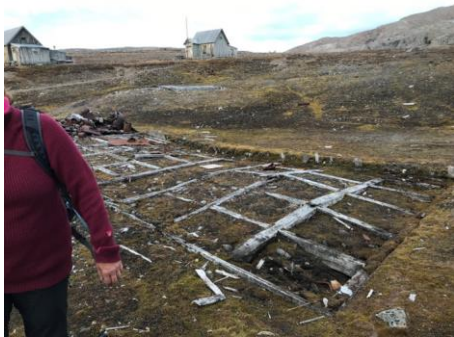
Figure 3. Foundation remains in Ny-London (2021), similar foundation type is believed to be used at Green Harbour House.
