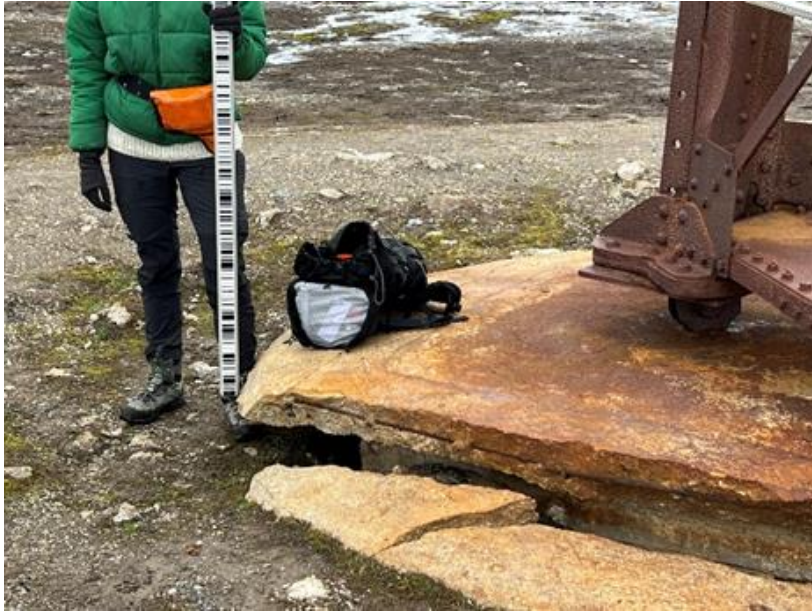
Figure 1. Terrain settlements (about 30-40 cm) around Luftskipsmasta (picture: 2022).
