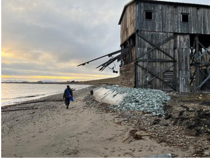
Figure 1. The Old cableway station (Taubanestasjonen) in Hiorthhamn protected by temporal solution against coastal erosion (picture: 2024).
