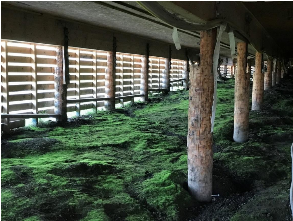
Figure 8: Pile foundation of UNIS Guest House, Longyearbyen. Picture: © Anatoly Sinitsyn/SINTEF AS.
