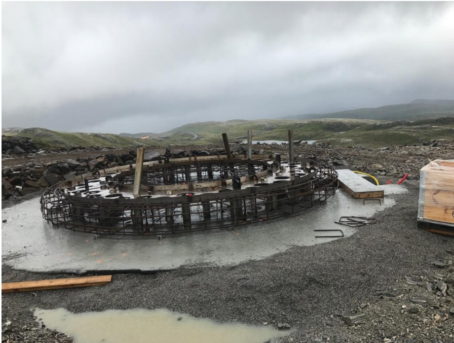
Figur 5. Fundament for turbin, Roan vindpark.
