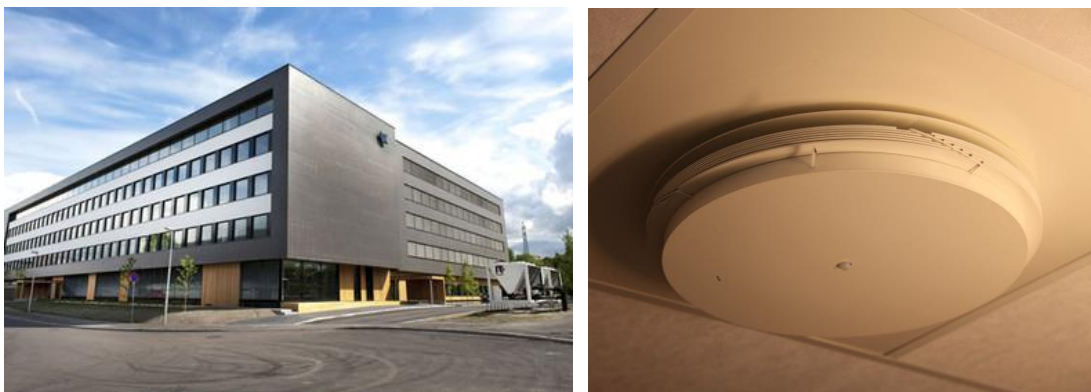
Figure 1. a) GK environmental building, Oslo. b) View of an active supply air diffuser.
