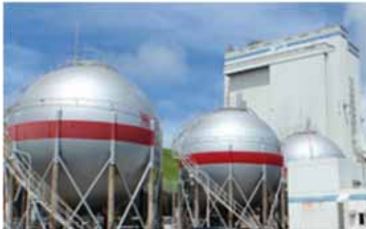
Storage tanks largest in Japan (Tanegashima rocket launch base)
