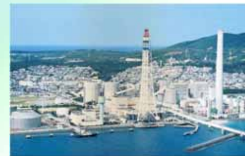
Energy plant (Coal-fired power generation plant)
