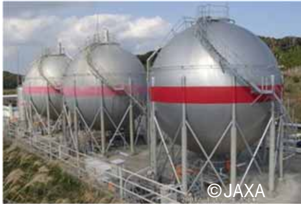
H-II rocket fuel hydrogen storage tank
