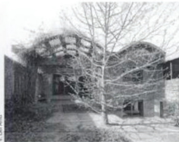
Fig. 7.22. Casa Dieste - enclosed courtyard.
