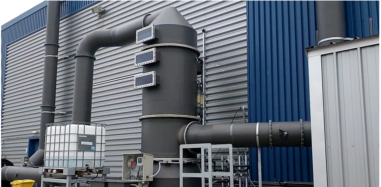
LCM has installed this 'wet-scrubber' to reduce any harmful emissions before they get exposed to the air.
