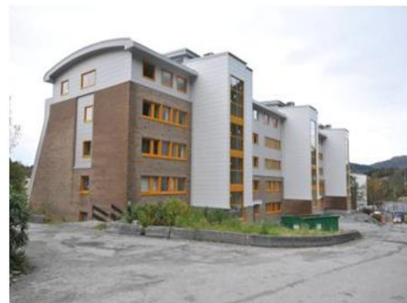
Fig. 5 After upgrading. Photo Jarl Høva
