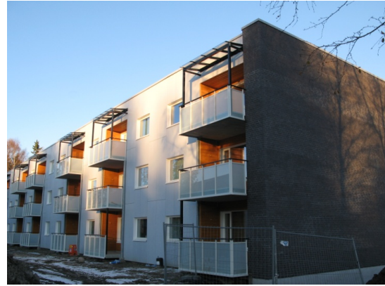
Fig. 3 After upgrading. Photo SINTEF Byggforsk
