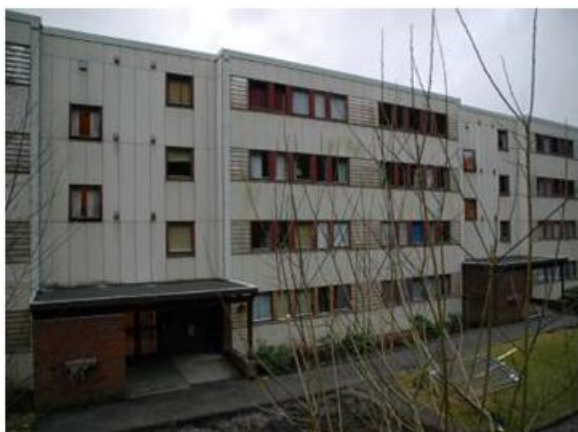
Fig. 4 Before upgrading. Photo Jarl Høva
