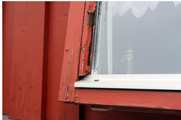
Figure 2. The façade is worn out, and the windows are in need for replacement.
