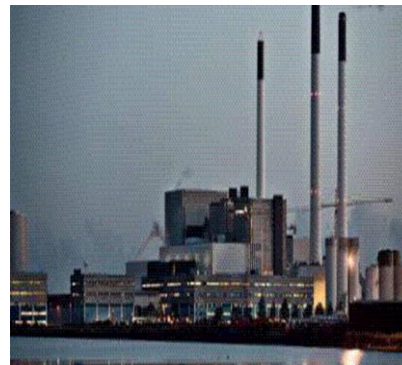
2012 Amager, Denmark 250 MW CHP
