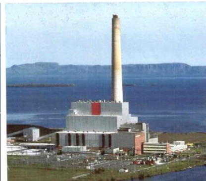
2013 & 2014 Thunder Bay, Canada 312 MW power station
