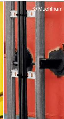
Mounting subsequent fixings with adhesive (instead of welding)
