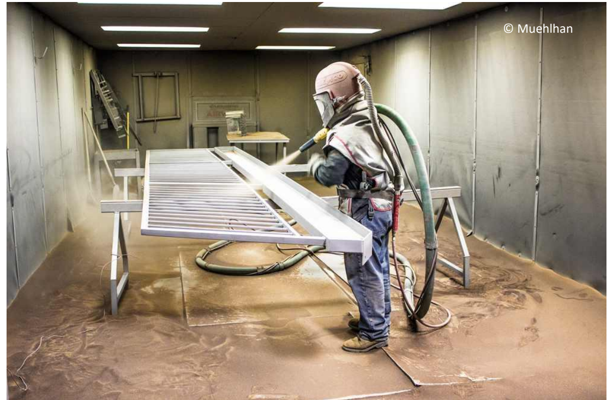
Garnet blast-cleaning of a part of an aluminum rail
