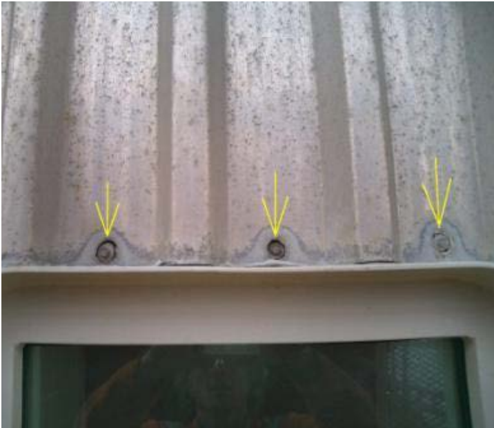
Under/around stainless bolts
