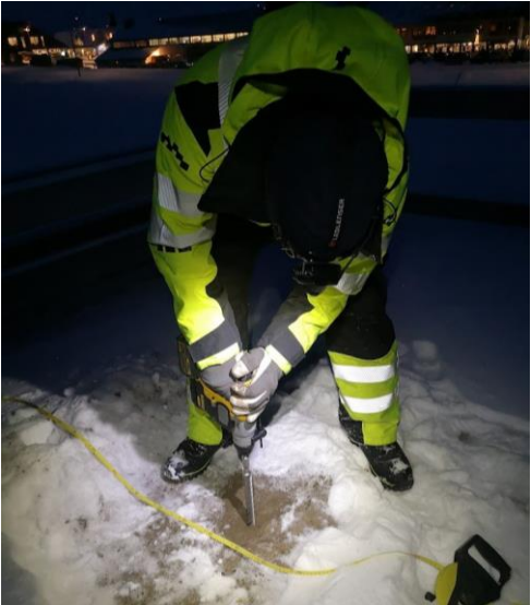
Installation of i-buttons. Picture: Enevoldsen, K. (winter 2022)
