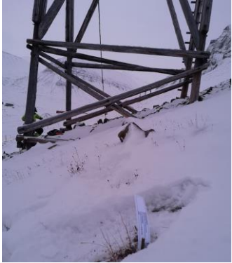
An i-button installed and marker with a shield. Picture: Enevoldsen, K.
