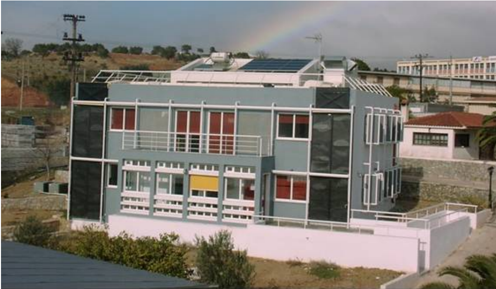
Picture 4: CRES Bioclimatic office building - south façade
