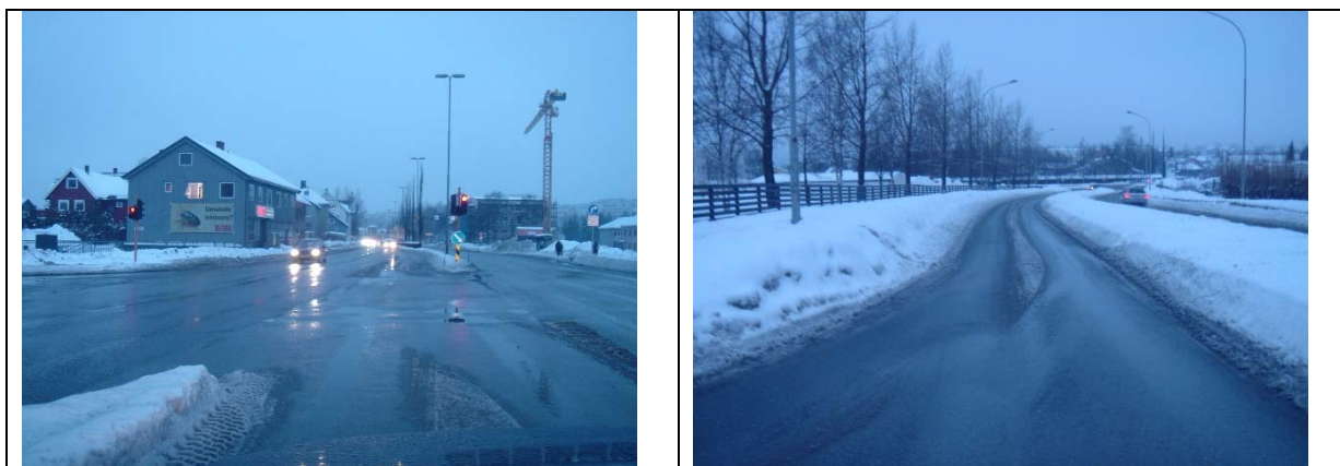
Figur 4.7: Bart i Holtermanns vei, men noe slaps mellom spor i Steindalsvegen
