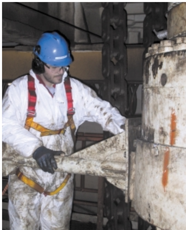
Installing risers demand high levels of security
