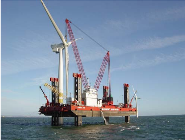
Figure 28: A jack-up barge used for installing offshore wind farms (Source: www.alternative-energy-news.info )
