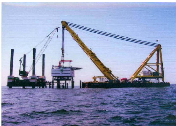
Figure 36: Installation of an offshore substation (Source: Deutsche WindGuard et al.)
