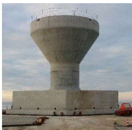
Figure 5: Gravity based foundation of the Nysted offshore wind farm (Source: www.nrc-cnrc.gc.ca )
