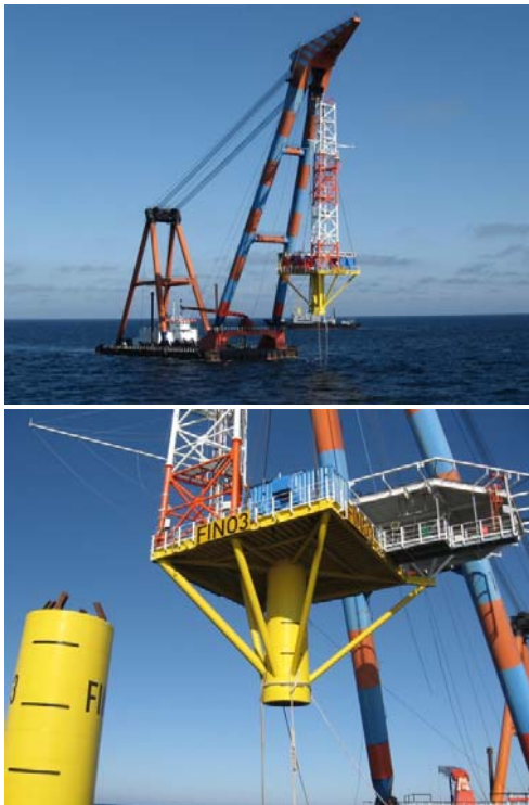
Figure 27: Construction of the met station Fino 3. Transport and installation of the platform with helideck and lower mast section (left). Construction of the mast (right) (Source: www.fino3.de )
