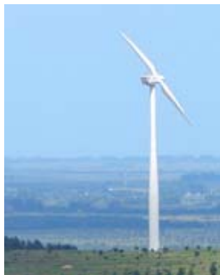
Figure 20: Two bladed wind turbine (Source: www.nordicwindpower.com )
