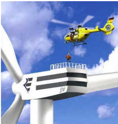
Figure 50: Landing on the nacelle by winching down from a helicopter (Source: Repower)
