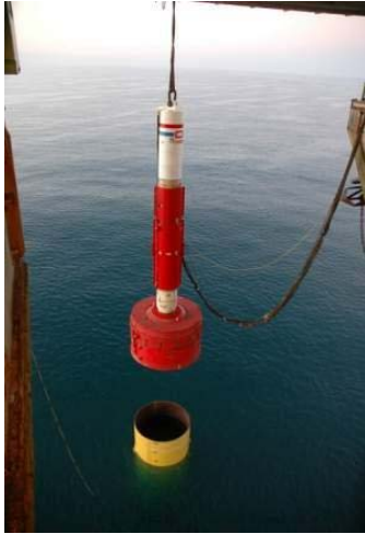
Figure 30: Hammer driving a monopile without anvil system (Source: www.nor-trade.dk )
