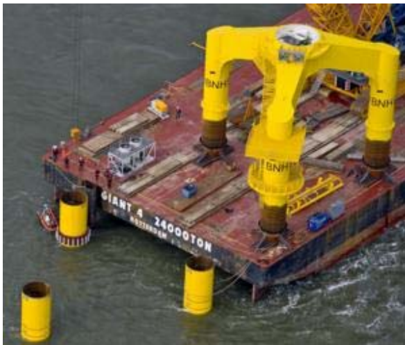
Figure 9: Tripile at the offshore wind farm Bard 1 (Source: www.bard-offshore.de )
