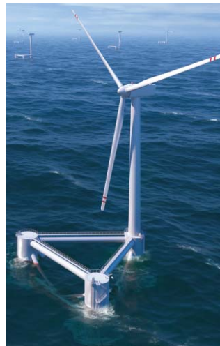
Figure 16: Windfloat concept (Source: www.principlepowerinc.com )
