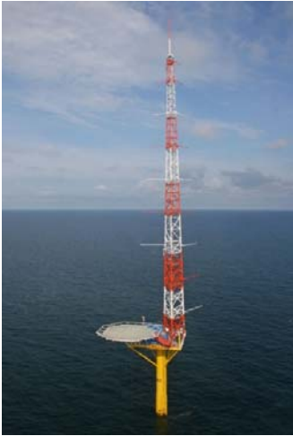
Figure 26: German met mast Fino 3 (Source: www.fino3.de )
