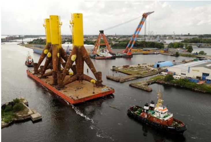
Figure 8: Transport of tripods for Alpha Ventus (Source: www.offshore-stiftung.de )
