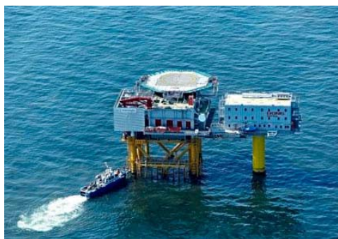
Figure 53: Offshore substation with accommodation platform alongside (Source: www.dong-energy.com )
