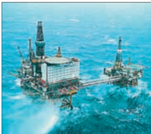
In 1987, water injection began from a well on the Ekofisk 2/4 K platform. The platform has a bridge connection to Ekofisk 2/4 B. The project was unique, since water injection to chalk formation reservoirs is unusual.
