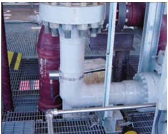
Field installation of a multiphase flow meter.
