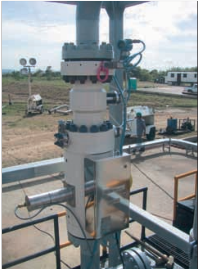
Sand meter SAM 400 installed on a production pipeline.
