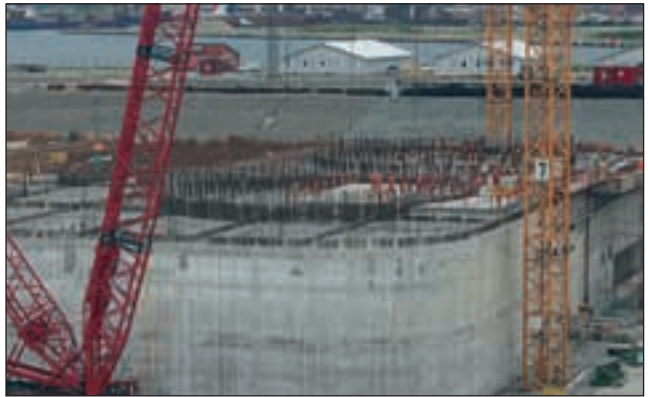
Enormous dimensions of the gravity base structure under construction at Sakhalin.
