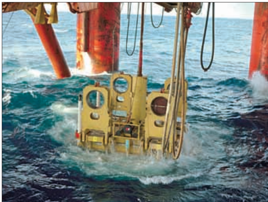
Installation of a HOST on the field. The wing elements have not yet been folded out after passage through the rig's moonpool.
