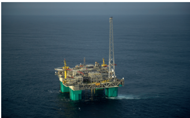
Figure 1. The Gjøa platform (Courtesy of GDF SUEZ)
