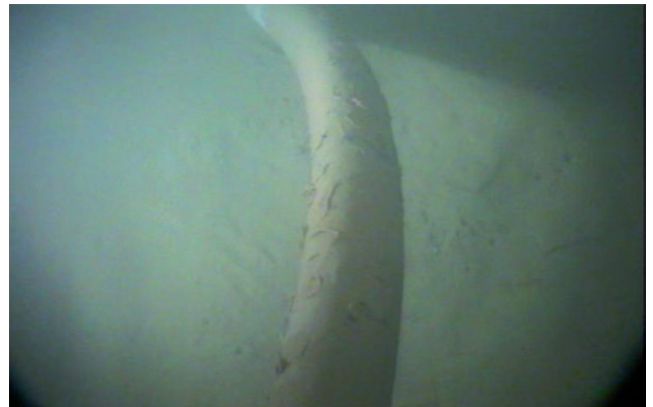
Figure 2. Upheaval buckling observed during the subsea inspection.
