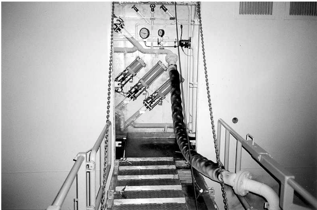
Figure 4 Close-up picture of the LNG filling station hatch at the shipside.
