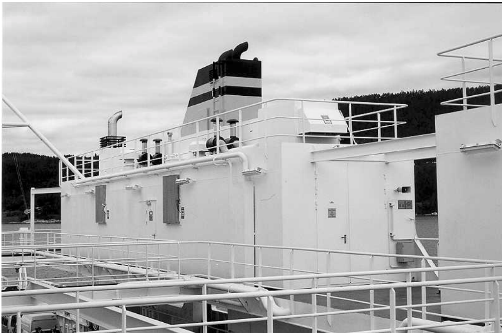
Figure 3. Two of the engine rooms separated by the main switchboard.
