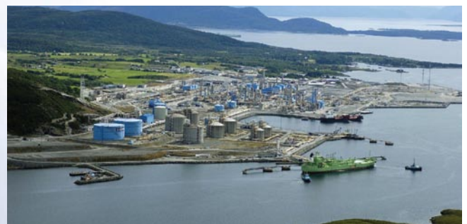
The Kårstø gas processing plant is a part of Gassled.
