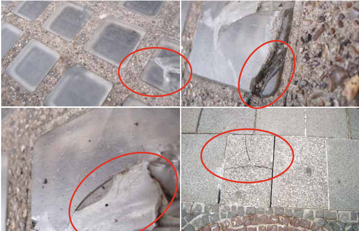
Figure 2: Example of a small natural stone pavement for a road and the damage.
