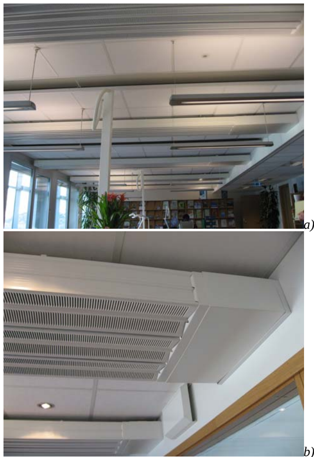
Figure C-10. Integrated ventilation and cooling in the ceiling elements, a) overview b) detail (photo Sintef Byggforsk / Matthias Haase)
