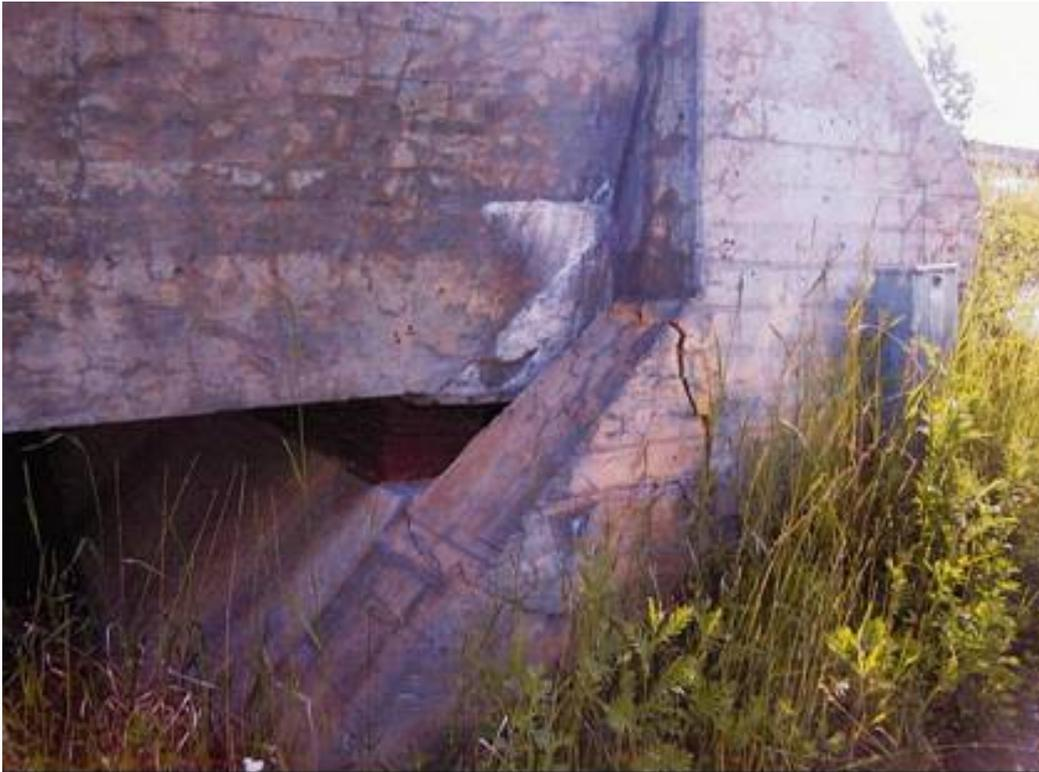
Figure 2.2-7: Norwegian concrete bridge. Due to expansion of the whole bridge plate, a major crack has occurred in the bridge abutment.
