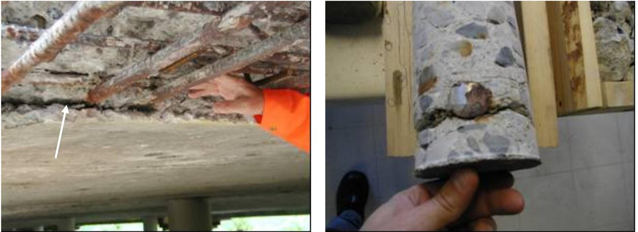
Figure 2.2-4: Delamination and cracking of a bridge deck where the primary cause of damage is AAR (same structure as the one to the right in Figure 2.2-3).
