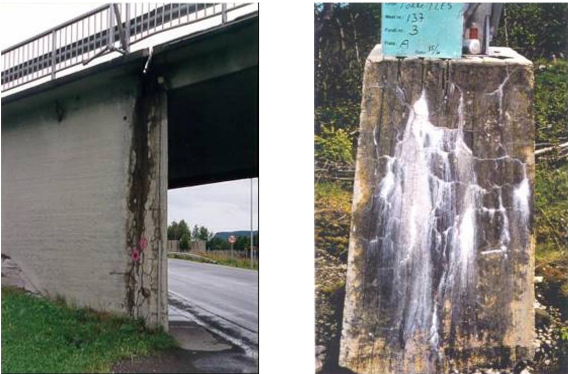
Figure 2.2-6: To the left: Concrete bridge in Norway. Draining water from the bridge deck flows down the concrete wall and set off the development of map-cracking in that area. To the right: Norwegian concrete foundation for high-voltage pylon exhibiting severe map-cracking due to AAR in combination with freeze/thaw damage.
