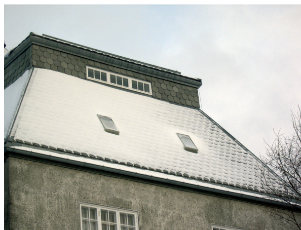
Figure 10. Even at very steep roof inclinations roof windows are covered by snow and ice. (Photo: SINTEF Building and Infrastructure)
