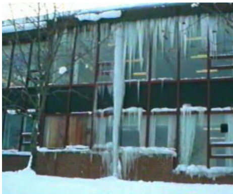
Figure 4. Large icicles in front of a school building's glass facade, representing a hazard to the children. (Photo: SINTEF Building and Infrastructure)
