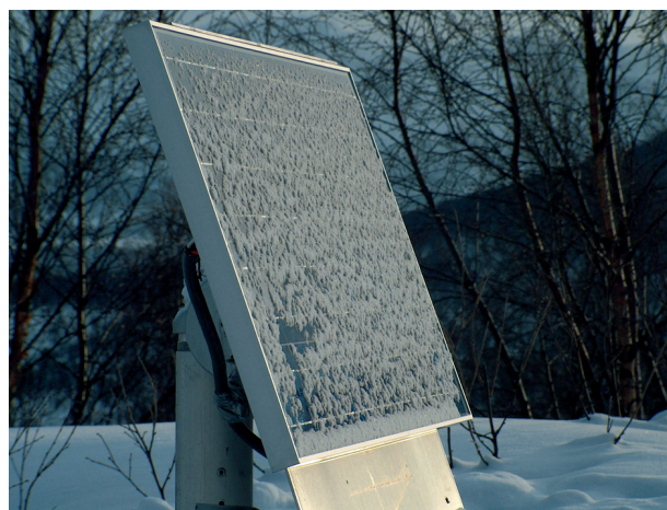
Figure 8. The inclination angle of this solar cell panel is as high as 70^\circ ; still the panel is covered by snow. (Photo: NTNU)
