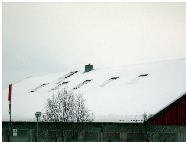
Figure 9. Roof windows covered by snow i.e. not fulfilling their purpose of letting daylight into the building. (Photo: SINTEF Building and Infrastructure)
