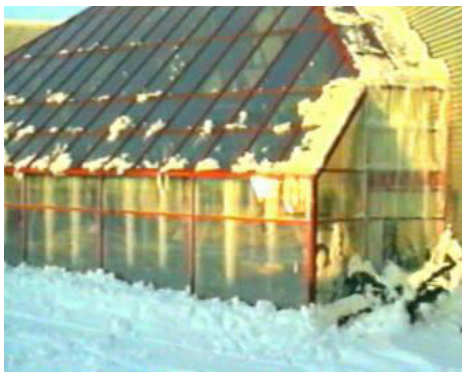
Figure 5. Large icicles covering a shopping centre's glass facade. To the right there is complete ice coverage. (Photo: SINTEF Building and Infrastructure)
