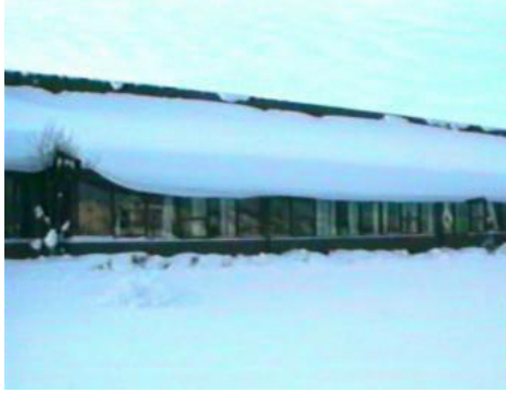
Figure 3. Snow from roof effectively covering the glass facade of a school building. (Photo: SINTEF Building and Infrastructure)
