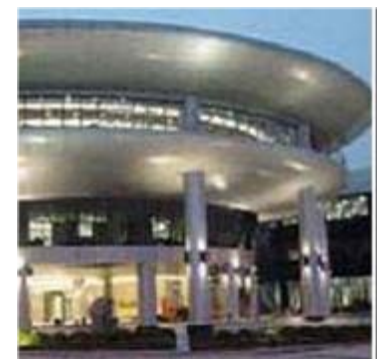
China Technology Center Shanghai, China
