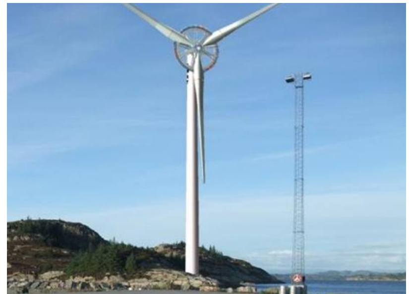
Concept: integration of generator with blades
