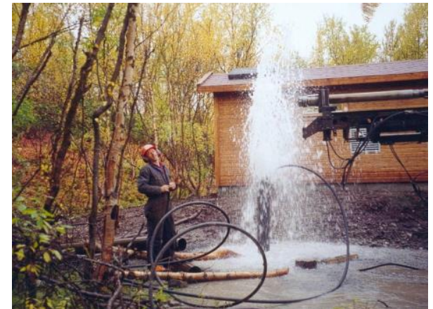
Ground water well drilled in gravel
