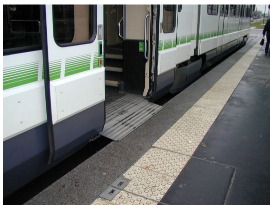
Varselflate langs perrongkant for lavgolvbuss i gågate.
