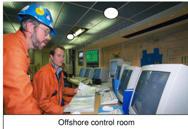
Offshore control room
