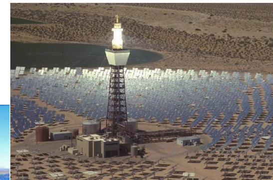
Fig. 3: Solar Power Tower System
