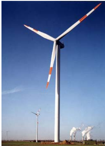
Prototype of 80 m tall Nordex 2,5 MW wind turbine located in Grevenbroich, Germany (Danish Wind Industry Association)
