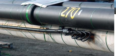
Installing of 18" DEH pipeline at the Orkanger test site.
