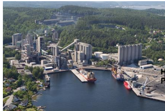
(NORCEM Capture Demo Project, large-scale project in planning Photo: NORCEM)
