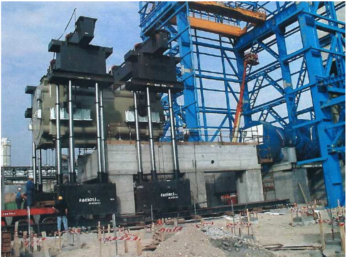
Figure 7-2: Installation with hydraulic gantry crane (example)
